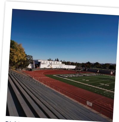
Diablo Valley College—Pleasant Hill The "Hall of Fame" entry and field house (far background) are part of the Kinesiology/Athletics complex construction.
