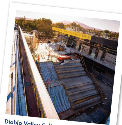
Diablo Valley College—Pleasant Hill The Art Complex is expected to achieve a LEED Gold rating.
